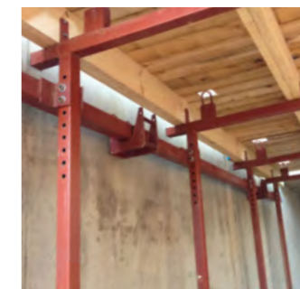
External Wall Platform Installation 外墙料台安装
