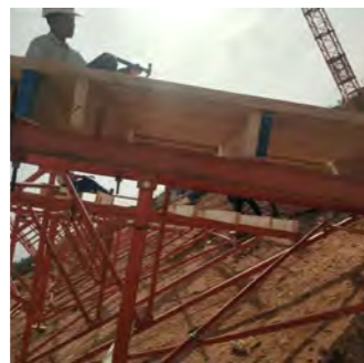
Operating Surface Installation 操作面安装
