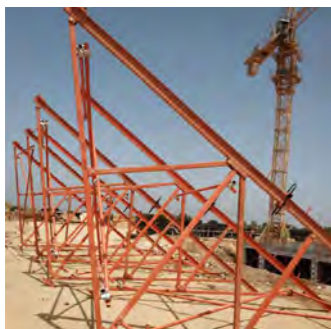
Steel Frame Installation 钢框架安装
