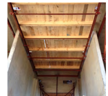
Stairwell Platform Installation 楼梯间料台安装
