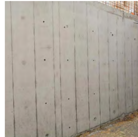
ALUMINIUM TUNNEL FORMWORK 铝制隧道模
