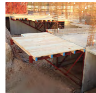
Opening Platform Installation 开间料台安装
